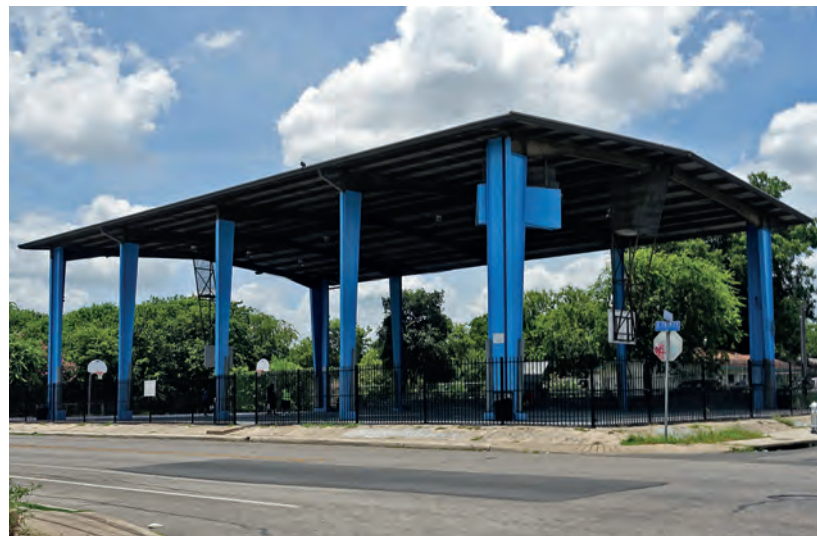
Fig. 5.8.6. The shade structure above this basketball court in San Antonio, Texas, USA, provides sun protection.
