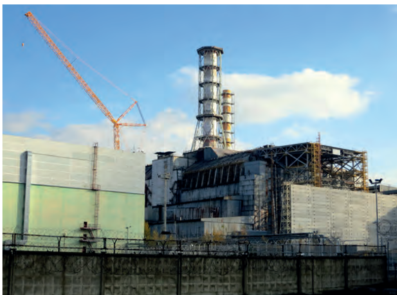
Fig. 5.18.2. The ruined reactor at the Chernobyl nuclear power plant in Ukraine. Exposure to radiation is the strongest known risk factor for papillary thyroid cancer.
