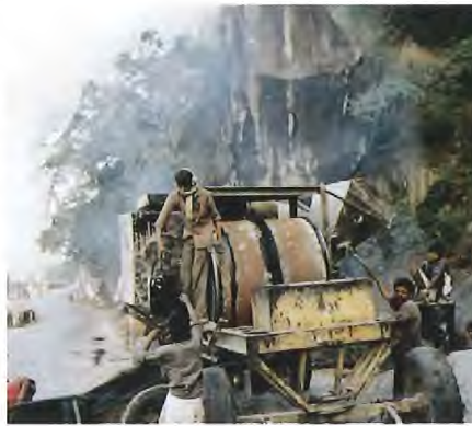
Figure 13. Work in road paving with asphalt can entail multiple exposures
