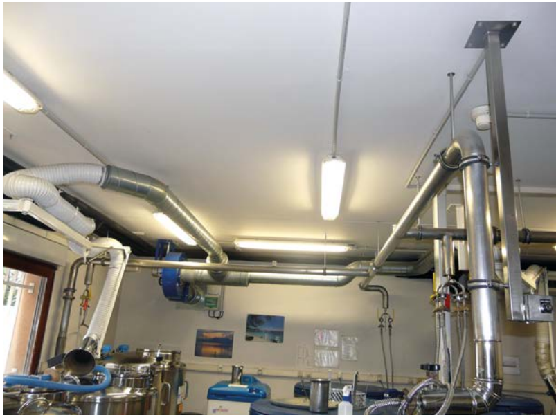
Fig. 18. Liquid nitrogen piping.
