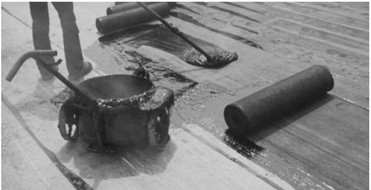
Fig. 1.4d Example of hot-applied bitumen (mopper)
