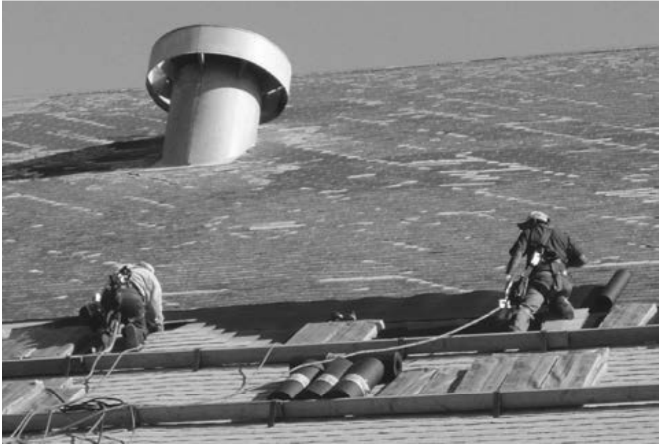
Fig. 1.4a Example of cold-applied bitumen
